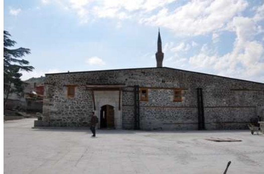
Figure 22. General View of Western Wall (Authors' Archive, 2015)
