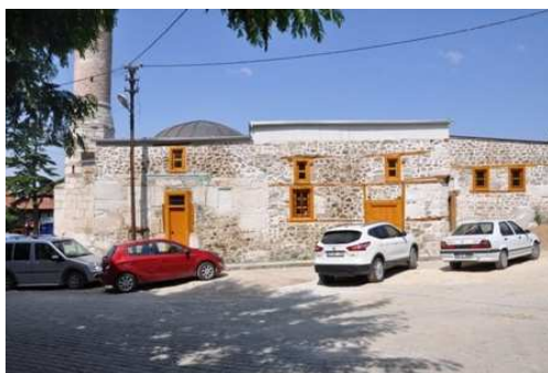
Figure 25. General View of Eastern Wall (Authors' Archive, 2015)
