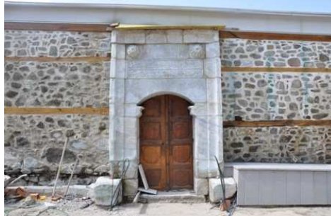
Figure 30. Door of Northern Wall (Authors' Archive, 2015)
