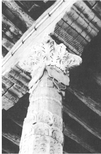
Figure 11. Use of Spolia Material on the Pole Bolster (Altınsapan, 1999: Figure 23)
