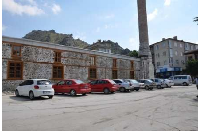
Figure 33. General View of Southern Wall (Authors' Archive, 2015)
