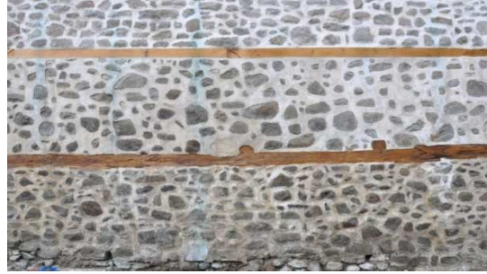
Figure 8. Use of Rubble Stone and Bonding Timber on the Main Wall (Authors' Archive, 2014)
