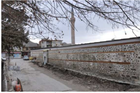
Figure 29. General View of Northern Wall (Authors' Archive, 2014)
