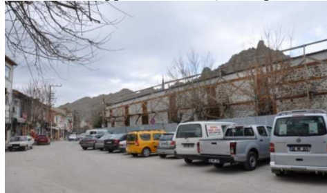
Figure 37. Restoration Implementation (Authors' Archive, 2014)
